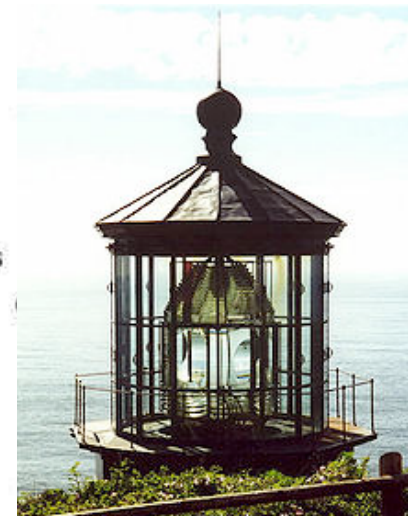
Cape Meares Lighthouse (Oregon); first-order Fresnel lens
